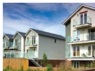
Rye Pottery, East Sussex. New residential development of town houses and flats on riverside location in historic town of Rye.
